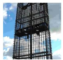
Cage Placement with O-Cell assembly Copyright © Fugro Loadtest 2010
